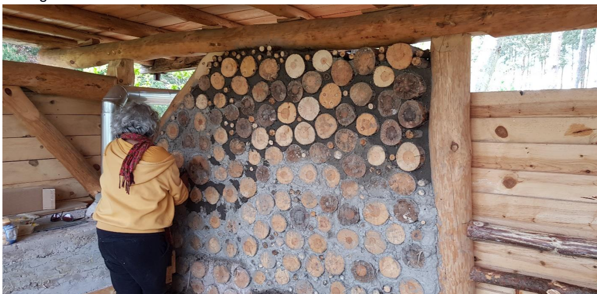
Putting the finishing touches to the earthen wall
