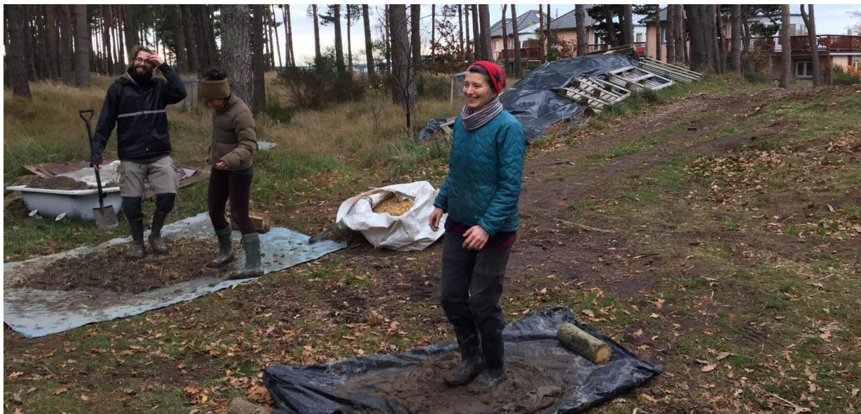
Mixing cob for the earthen elements
