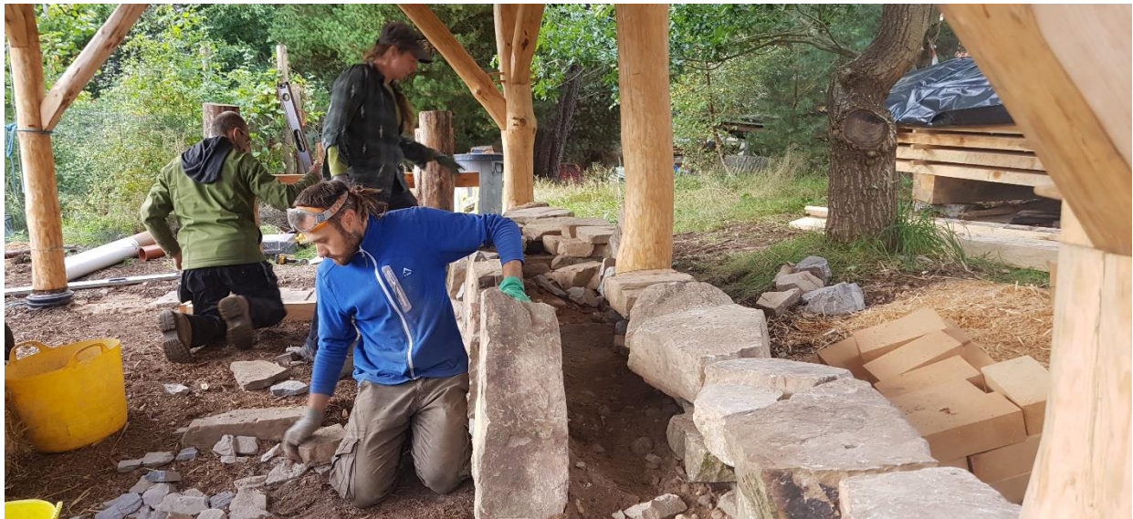
Building the foundations for the heated earthen bench.
