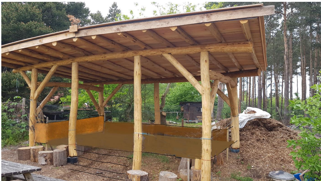
The round pole timber frame with the sketching in of where the floor, bench and stove would be located. Before this phase of construction began.
